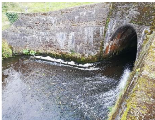
Plate 3-2 Blackwater (Clare) River – view of steep slope with fish pass on culvert beneath Ardnacrusha Headrace Canal (18/09/2022)
